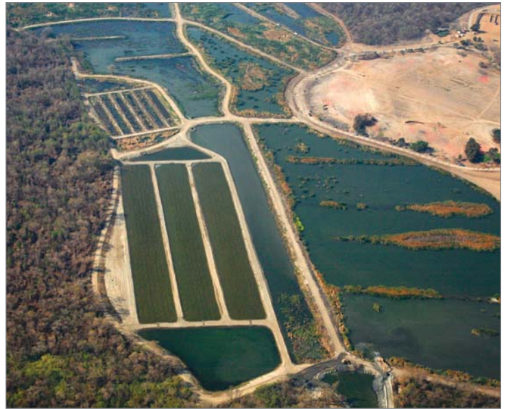
Figure 7: The open water unit process cell at the Prado Wetlands. Photo courtesy of Scott Nygren, Orange County Water District.
