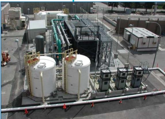
The Groundwater Replenishment System's microfiltration process consists of a 6-mgd USFilter CMF-S submersible system. This process is a smaller-scale version of the 86-mgd microfiltration facility currently under construction at the same site.
