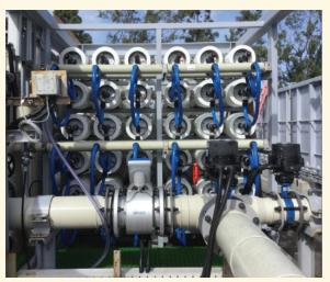
The City is experienced with recycled water and advanced membrane treatment, through the successful implementation of non-potable reuse and seawater desalination (shown here).
