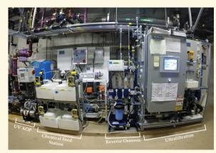
An image of the 1 gallon per minute PureWaterSF DPR pilot project that was used to research decentralized DPR and provide public tours.
