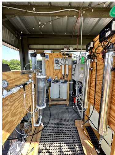
Photograph 1 – Complete AWP train deployed at the DPR Pilot Site at the City of San Marcos WWTP
